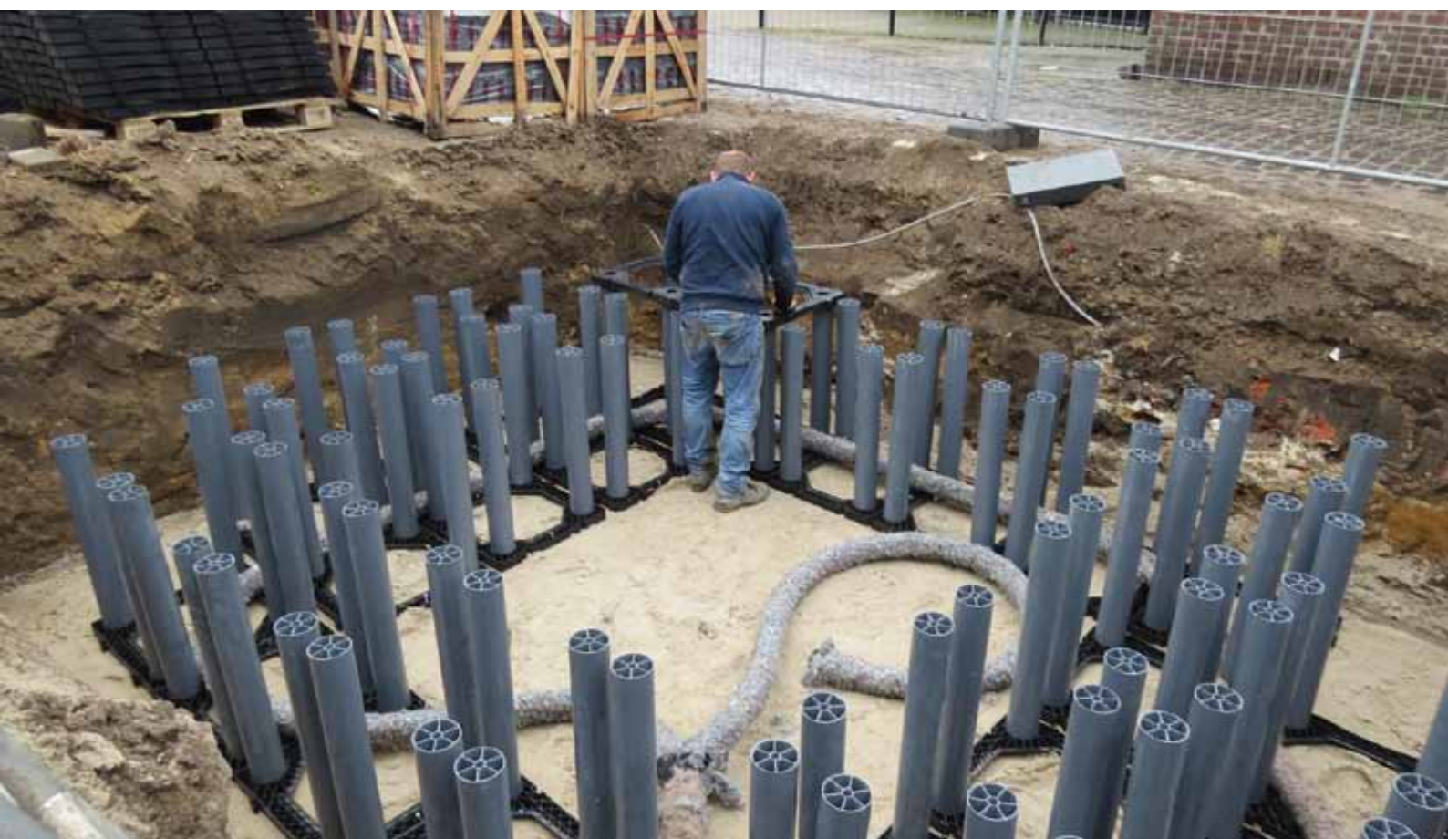
Boombunker in aanbouw in Venray.
